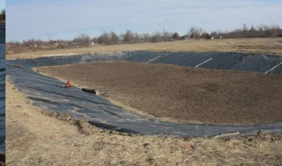
MRPTS vertical flow bioreactor, before flooding, fall 2008
