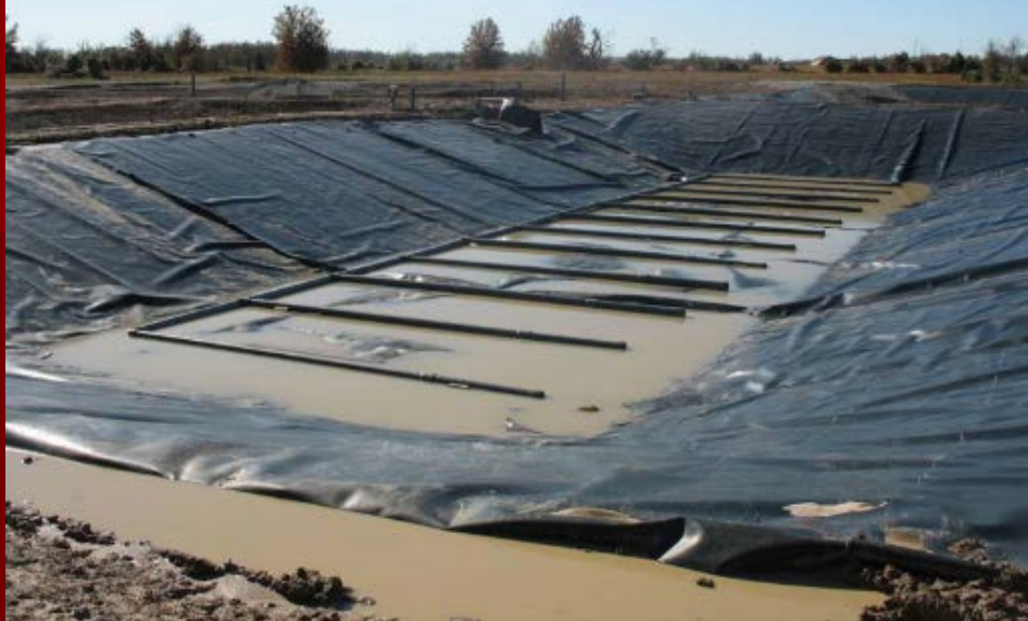
MRPTS vertical flow bioreactor, under construction, fall 2008
