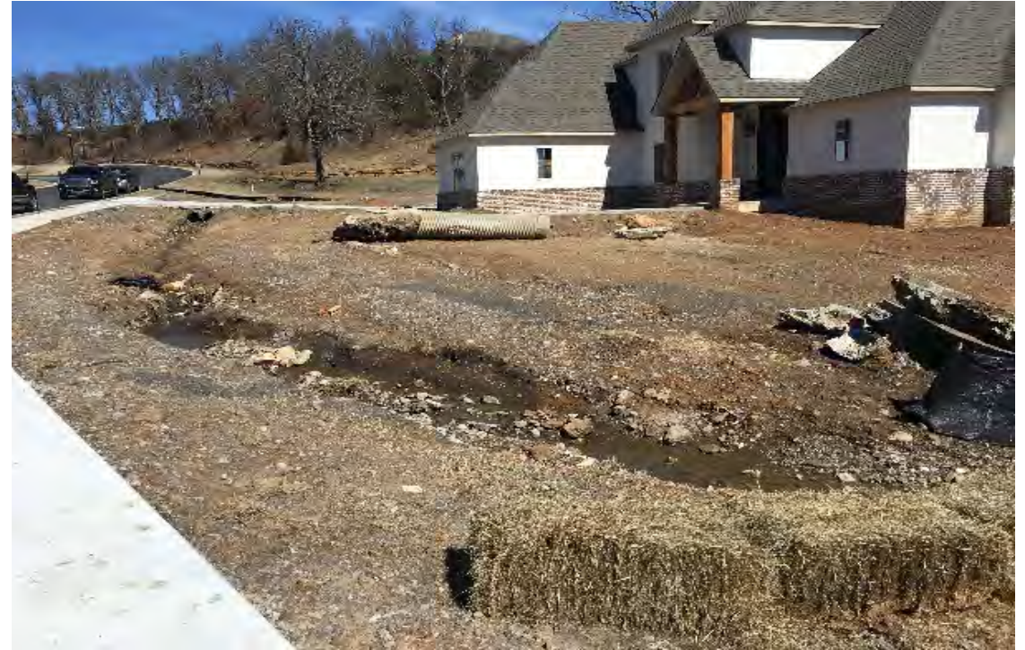
During construction – lack of erosion control
